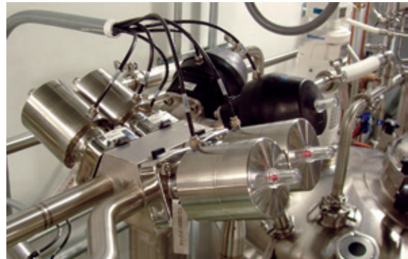
Images of the installation
